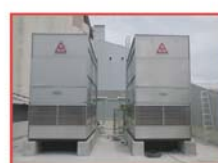
ENCLOSED TYPE / EVAP.CONDENSER
